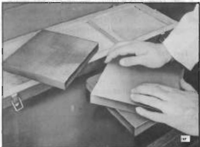
Fig. 2 - Refinishing Lapping Blocks
